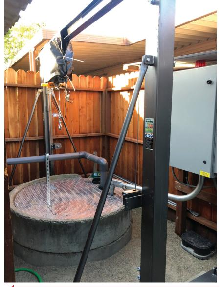
The pump station includes our 3" Shinmaywa CNWX pumps on rails, gastight hatch cover, bronze swing check valves and sch 80 pvc piping with ball valves. The control panel converts 230V single phase to three phase using VFD's with 4 float functionality and an alarm dialer. The owner stepped it up by connecting the system to a generator so it has power during PG&E blackouts.
