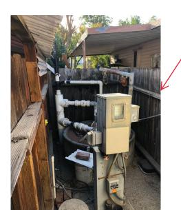
The picture to left and the one on the upper right corner were taken from the same spot. This pump station no longer has odor issues, Shinmaywa pumps will not clog on a daily basis and the controls were moved over to the left of the pump station yard area to create space for the gantry.
